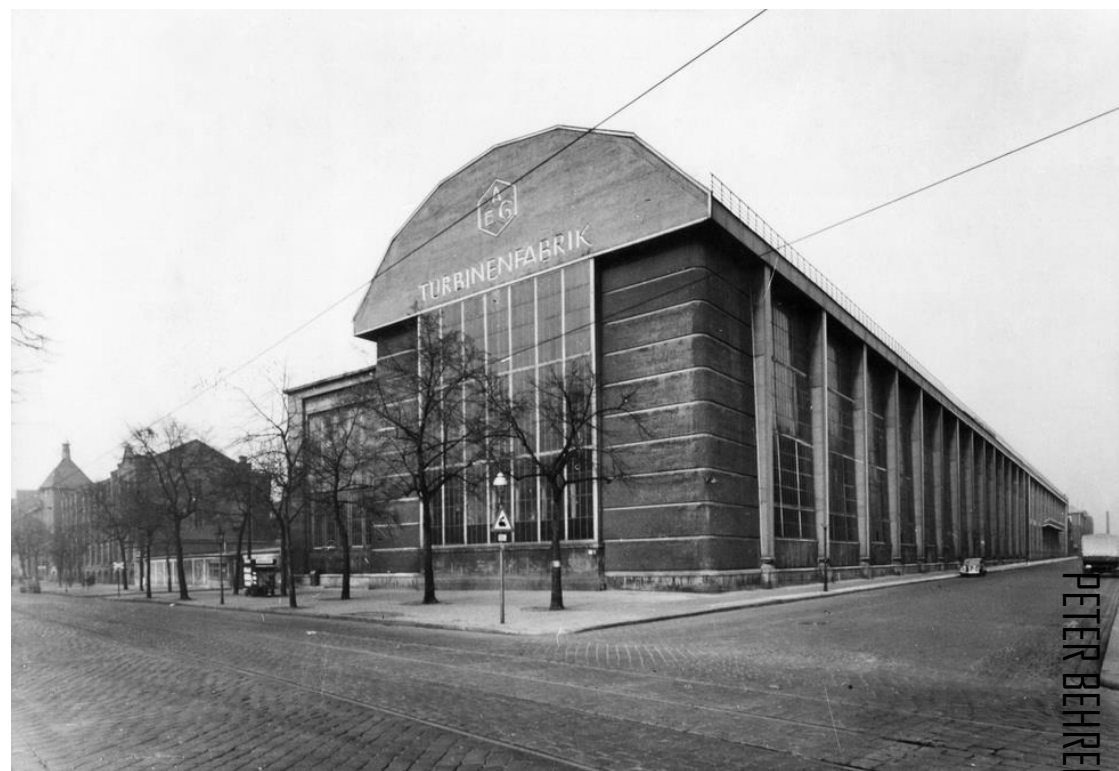
aeg turbine factory in Berlin, built by peter behrens in 1909. © Getty Images
